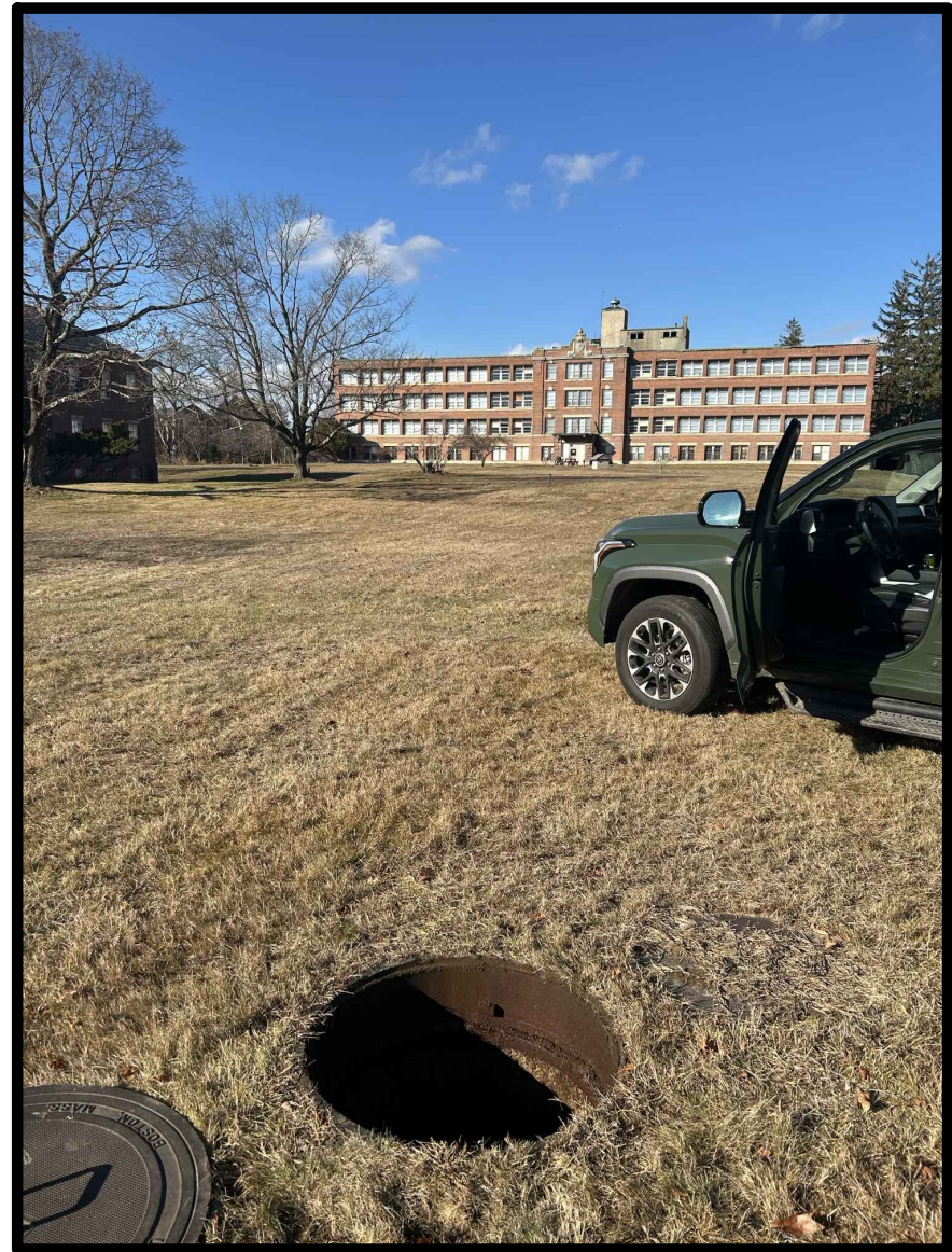
TYPICAL VIEW ABANDONED STEAM LINE MANHOLE 1
