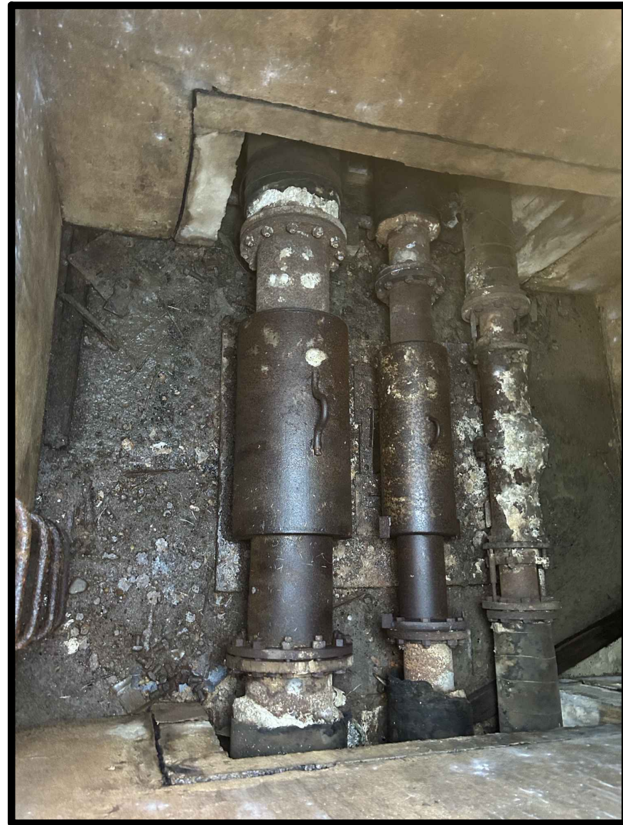
TYPICAL VIEW INSIDE MANHOLE OF ABANDONED STEAM LINES 3
